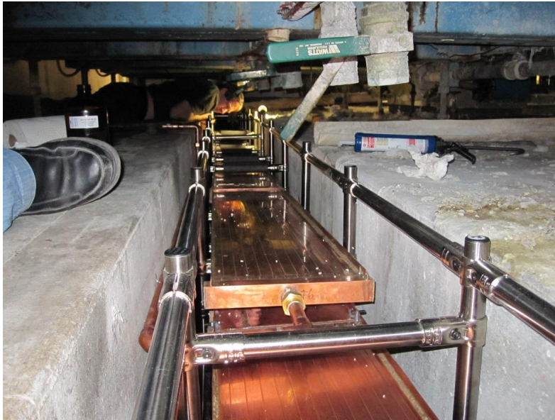
Image 2 – Ecodrain M1000 Heat transfer panels being installed beneath conveyor washer
